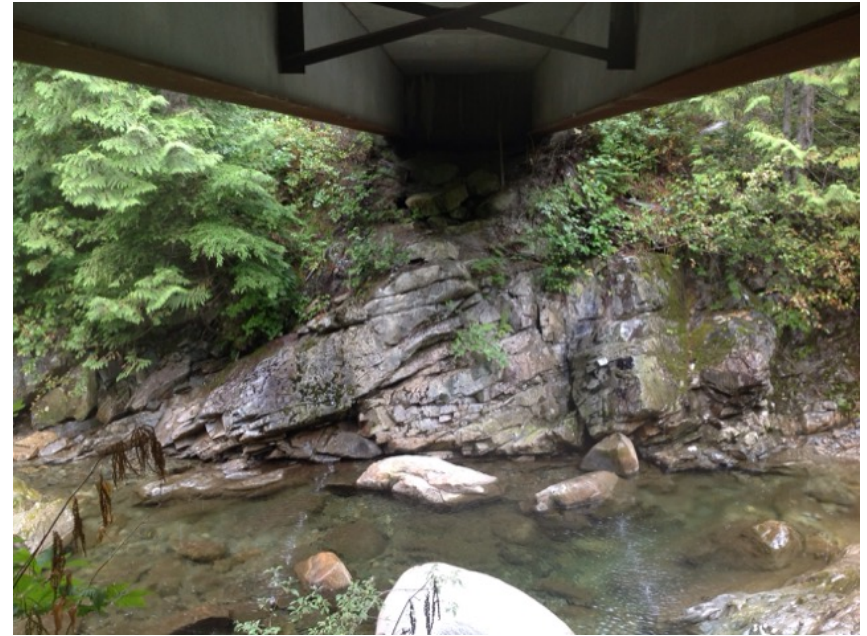
Right Bank Abutment when facing downstream
