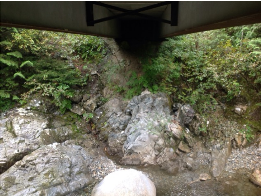
Left Bank Abutment when facing downstream
